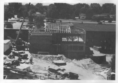
Marquardt Village's new Karl Fischer Activity Center is rapidly being built. Roof trusses were being placed when the above picture was taken. Inspecting the progress being made (below) are Marquardt executives Boyd Flater and Milo Loppnow.
