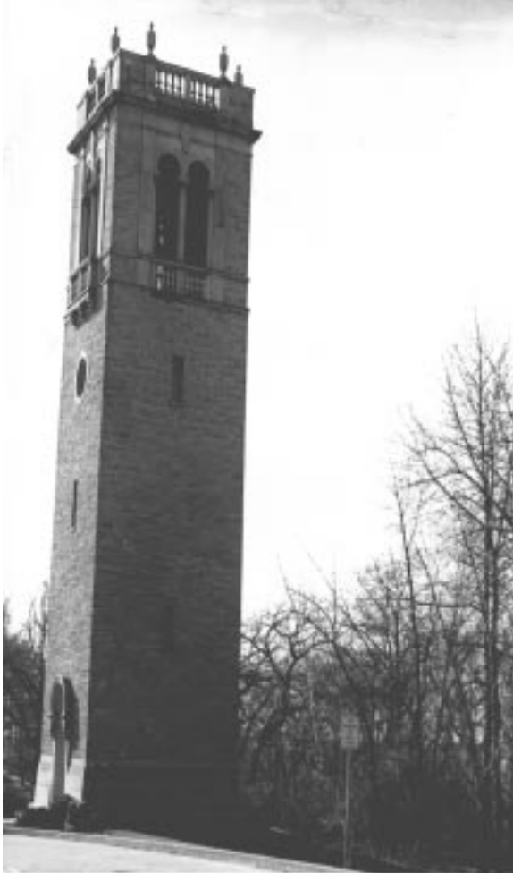
Fig. 1. The carillon tower c. 1938. [Series 9/1, Carillon, jf-57]
