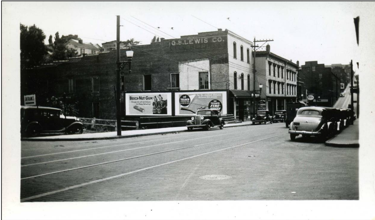
FIGURE 8. G.B. Lewis Company Branch building, Lynchburg, Virginia ( Courtesy of Lynchburg Museum System ).
